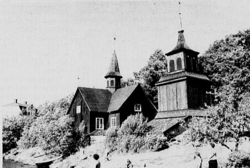
Fagervik church and bell tower, with manor house on left
