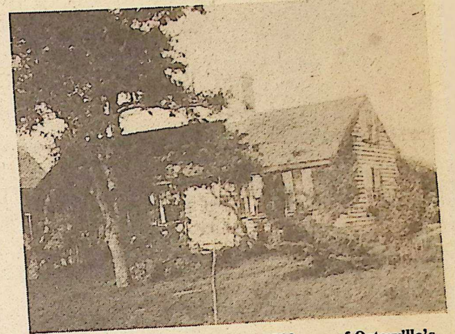
The old Cammett House, circa 1728, one of Osterville's oldest houses, is threatened to be torn down unless the Osterville Historical Society can raise the funds needed to move and restore it. (Photo courtesy of Paul Chesbro)
