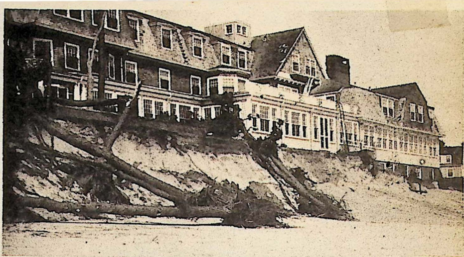
This photo, taken from the beach, shows the damage sustained by trees, beach and the Wianno Club itself after the 1944 hurricane.
