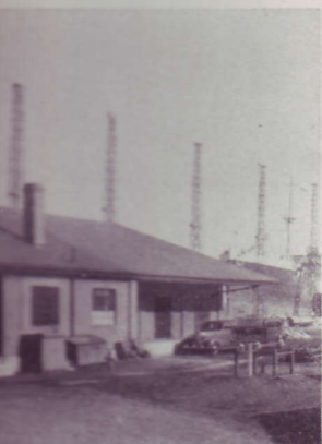
marine terminal WPA workers reconstruction building, recondi- and laid new concrete the river front
