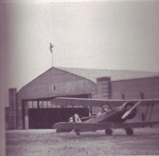
WPA workers rebuilt the hangar and added administration building at Little Rock
