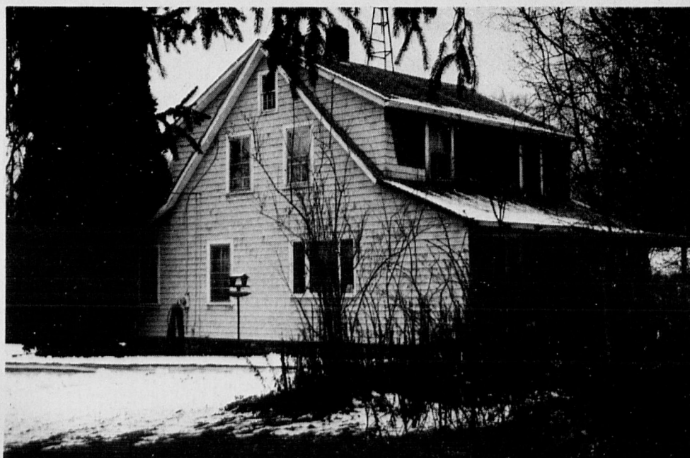
Kurikka's house in North Stonington (CT). Some wings and dormers have probably been added. 1998 photo by Burton Jernström.
