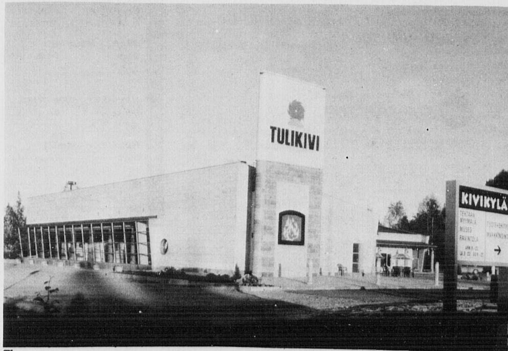
The new corporate complex of Tulikivi Oy with the research and development wing on the left.
